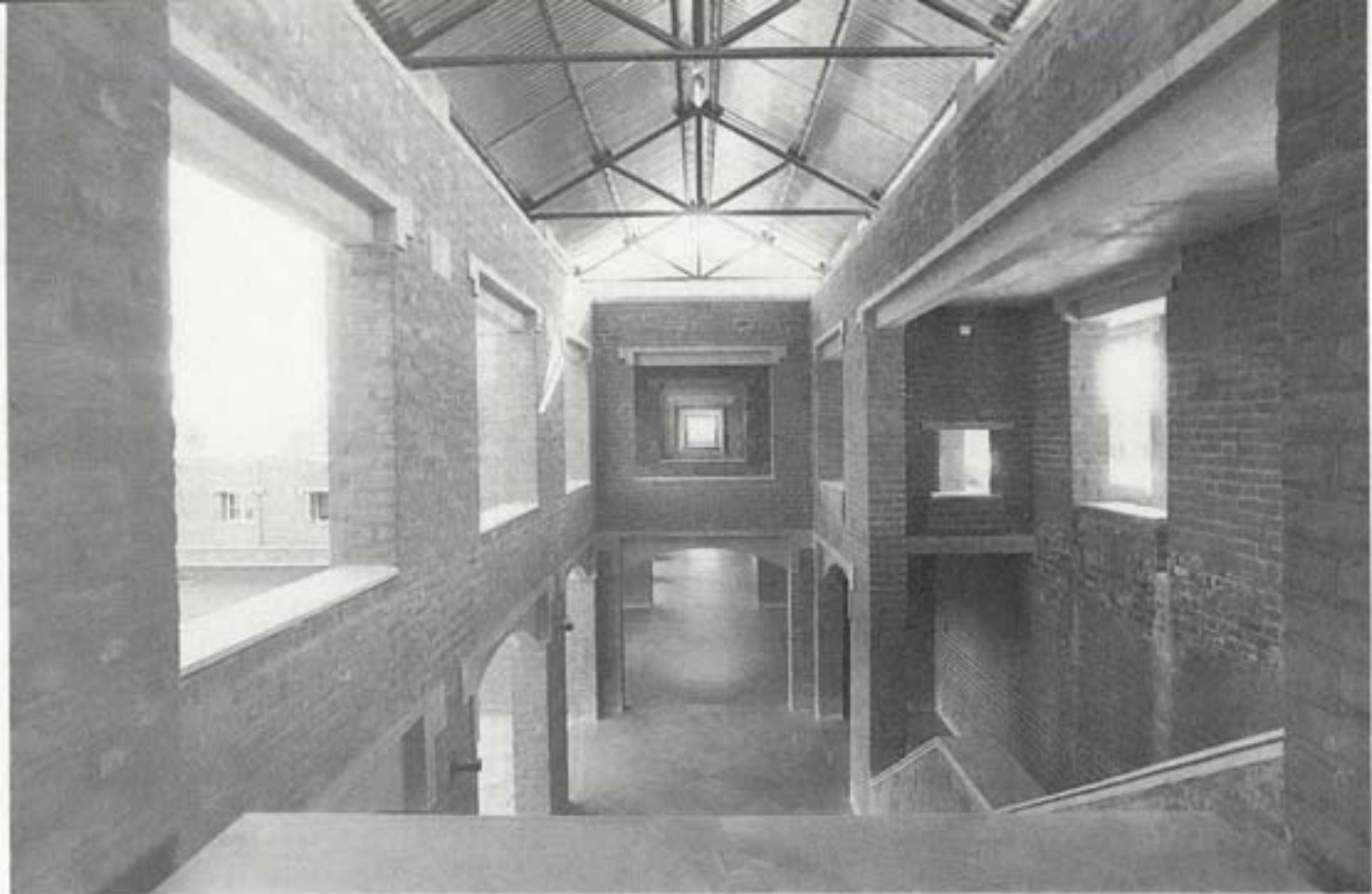
View of the main corridor
