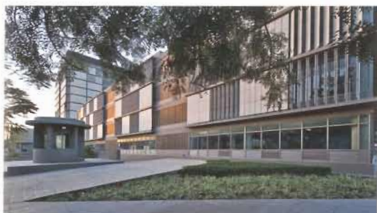
the façade system of aluminium framed sliding windows screened on the outside by vertical louvers.
