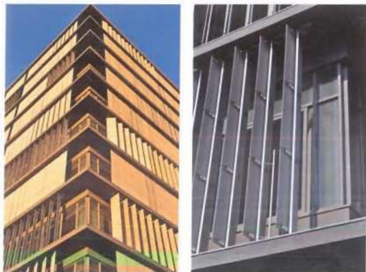
the detailing of the windows.
