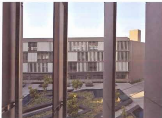
the louver system limits glare, ensuring visibility from the interiors.
