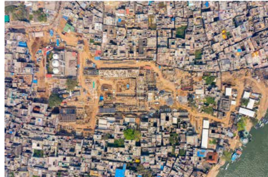
Drone shot of the project under development
