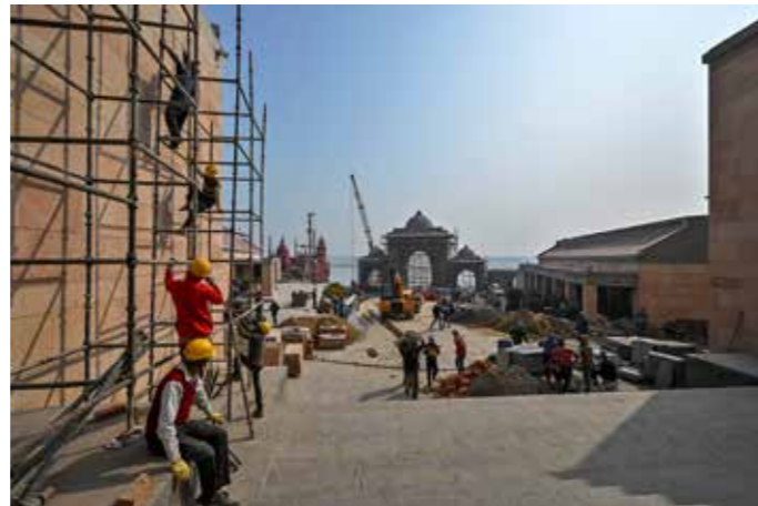
The pathway from the Temple to the Ganges, under construction
