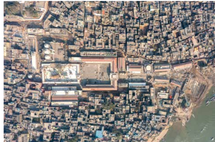
Drone shot of the project nearing completion
